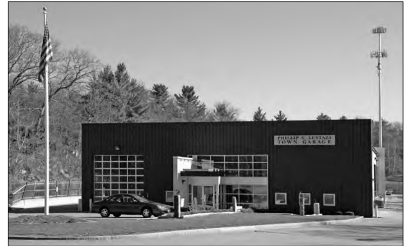
The Phillip S. Luttazi Town Garage. Photo by David W. Stapleton.
